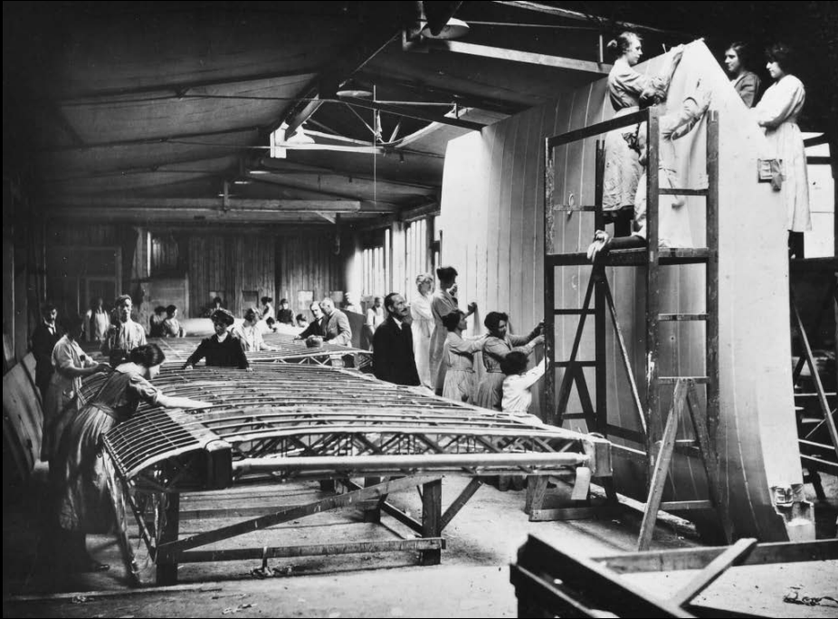
Aircraft Wing Building during WW1
